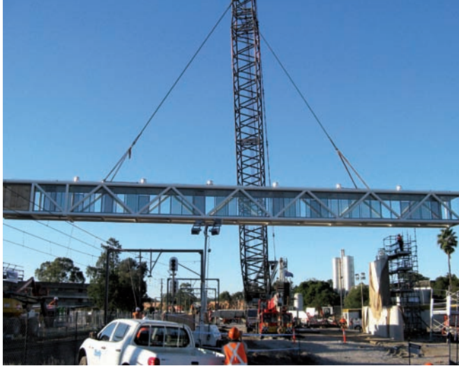
Construction zone: putting a walkway in place at Liverpool Hospital
